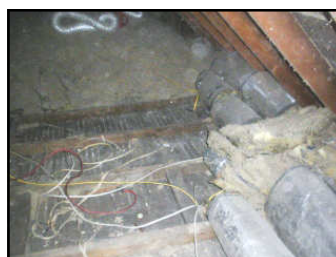
Vacuum before laying rolled insulation back.
