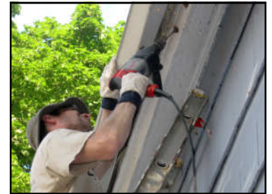
Installing Soffit Vents
