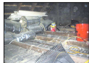
Vacuum before laying rolled insulation back.
